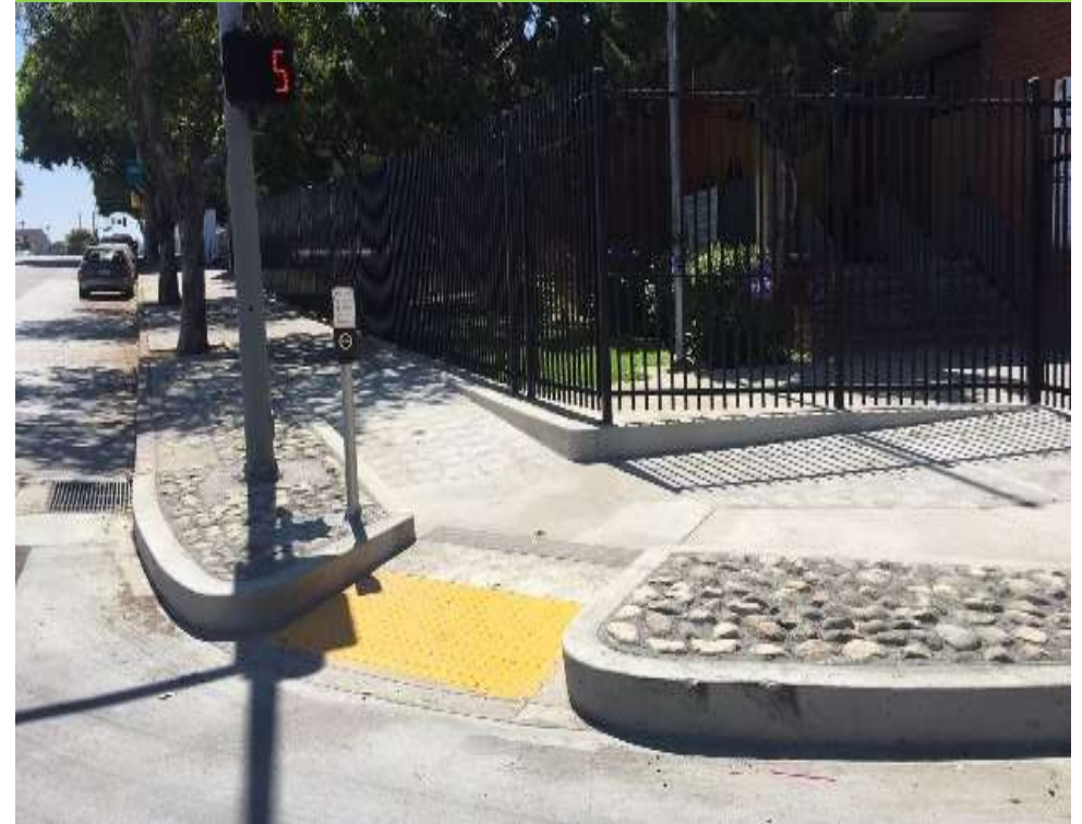
After at Temple Blvd. and Douglas St.
