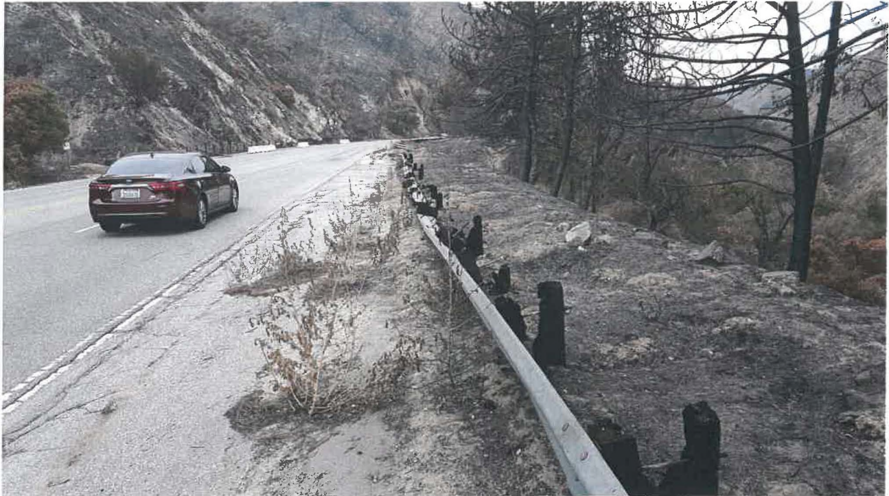
Photo 2: View west along the north side of La Tuna Canyon Road. Note the burnt-out wood support posts for the guard rail.
