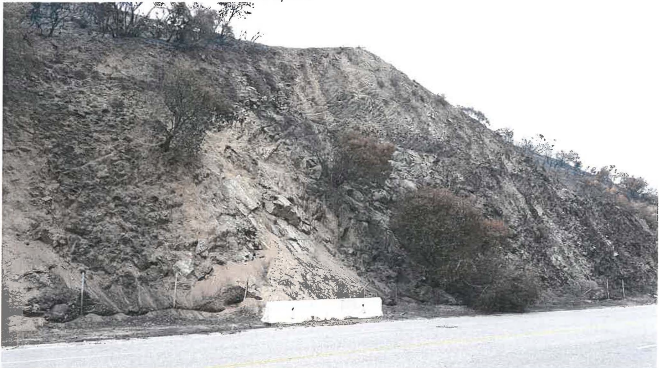
Photo 5: View south towards an active debris and rubble apron that has overwhelmed a 'debris fence' that consists of standard chain link.
