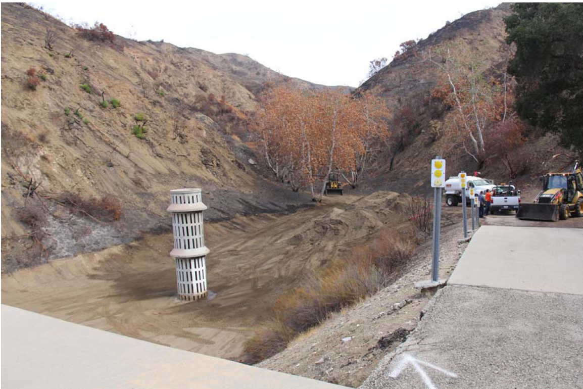
Site 4: Debris being removed from behind the Chandler Debris Basin.
