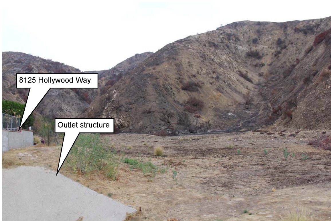
Site 3: Looking north across a debris basin located adjacent to the property of 8125 Hollywood Way. Note the amount of debris that has accumulated in the basin.
