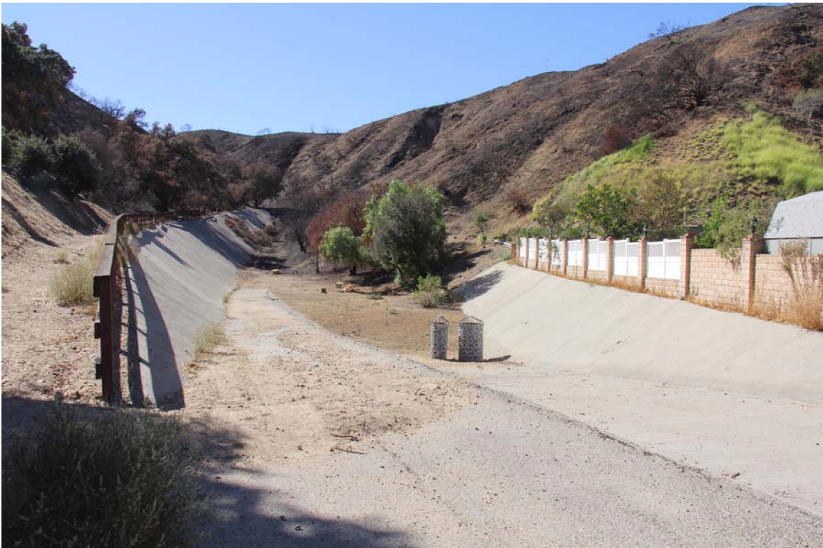
Site 5: Looking southwest towards a concrete-lined debris basin located on Santa Monica Mountain Conservancy property, which is located immediately adjacent to 8945 Morning Glow Way.
