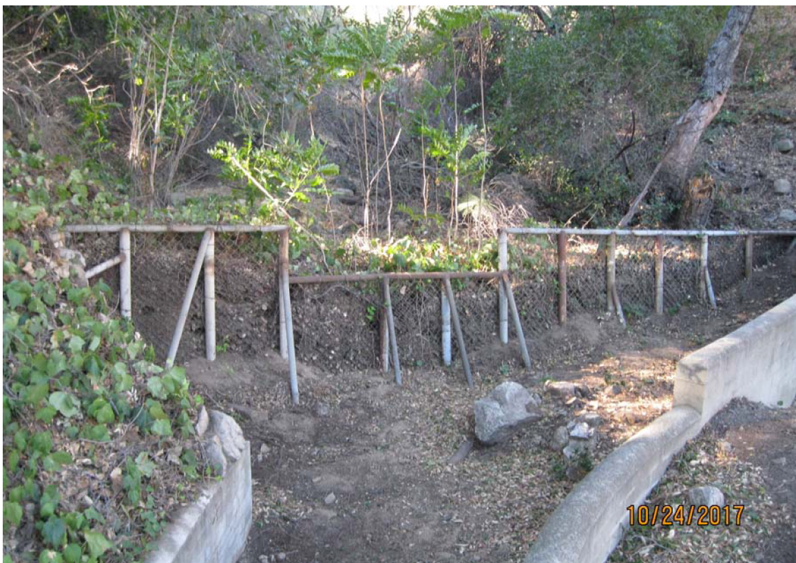
Site 16: Looking southwest towards the debris fence that is located west of the McGroarty Cultural Center Building. Note, the accumulations of soil and debris behind the debris fence.
