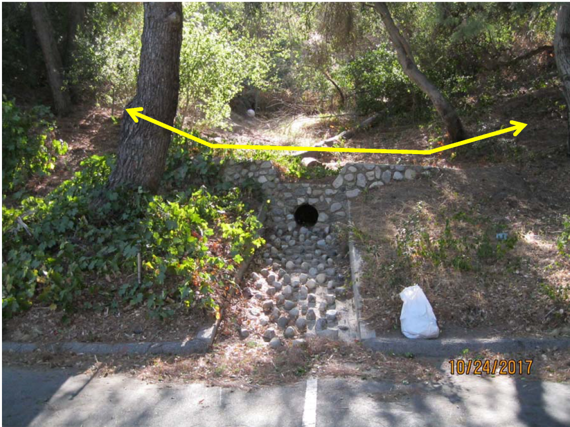
Site 16: Looking south towards the stacked cobble and mortar-filled catch basin. The double yellow arrow points out where a 40' (L) and 4' (H) debris fence has been recommended to increase debris storage capacity and prevent the catch basin from clogging.
