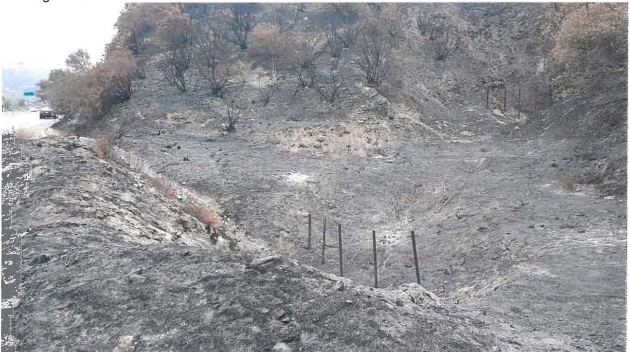
Photo 3: View east from the shoulder area next to a culvert along the south side of La Tuna Canyon Road. Note the two debris fences.
