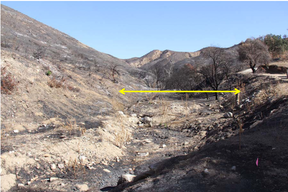
Site 8: Looking southeast and up Teazole Canyon which has been severely burned. The double yellow arrow points out where a revetment or debris rack has been recommended to be installed across the channel.
