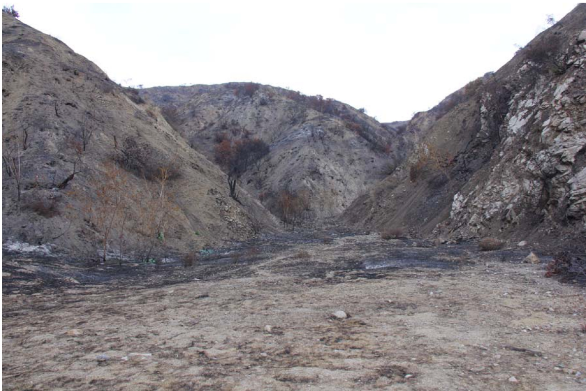
Site 3: Looking north and up the drainage which empties into the northern end of the debris basin. Note the amount of accumulated soil and rock in this portion of the basin.
