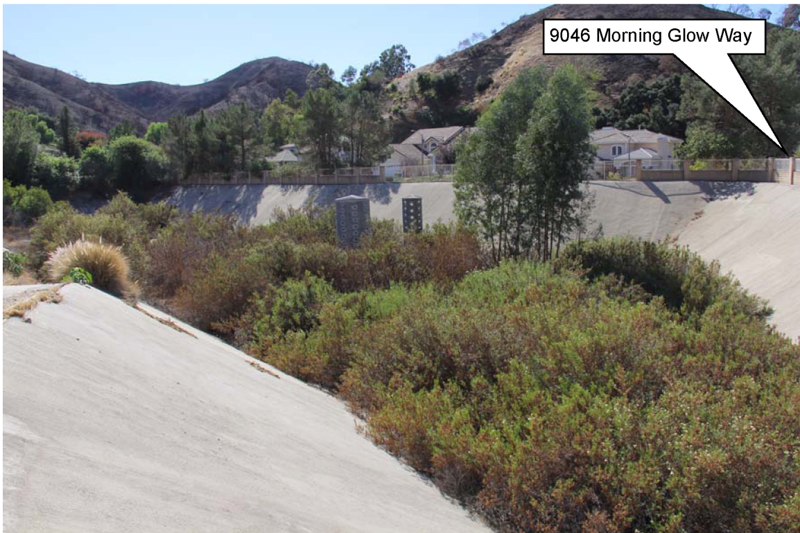
Site 6: Looking southwest across the debris basin. Note how the basin is overgrown and clogged with vegetation.
