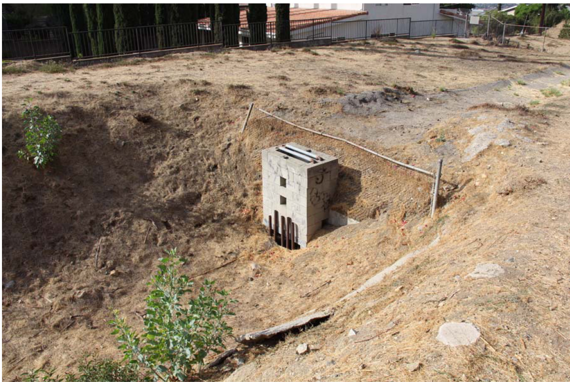
Site 2: Close up of a concrete block outlet structure located at the eastern end of the drainage swale.
