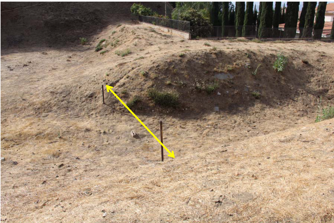
Site 2: Looking south across the channel leading to the outlet structure. The double yellow arrow points out where a 25' (L) x 10' (H) revetment or debris rack has been recommended to be installed across the channel to prevent the outlet structure from becoming clogged with debris.
