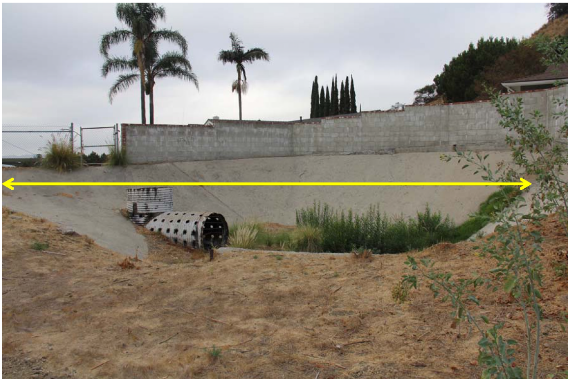
Site 3: Looking west towards the outlet structure. The double yellow arrow points out where 65 linear feet of debris fencing has been recommended to be installed in order to prevent the outlet structure from becoming clogged with debris.
