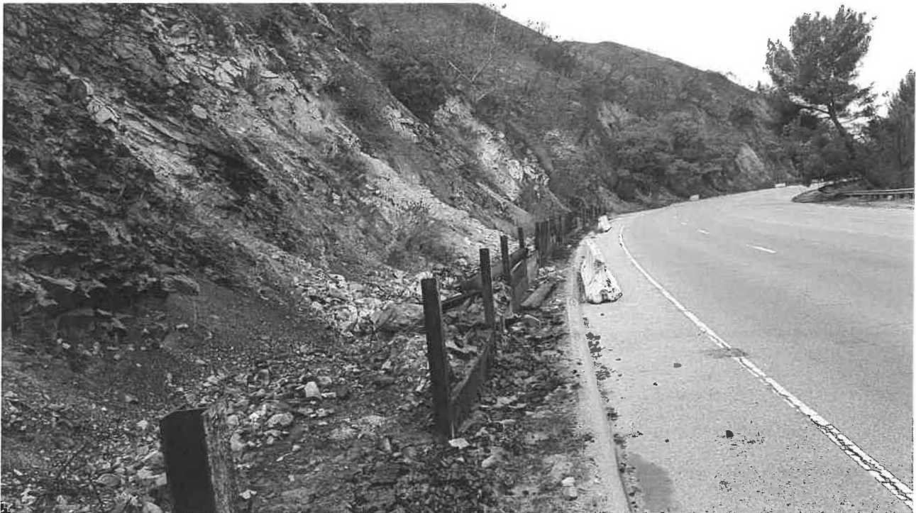
Photo 1: View west along the south side of La Tuna Canyon Road. Note the sections of lagging that are completely burnt out as well some sections that are relatively intact. Also note the debris piles behind the slough wall.
