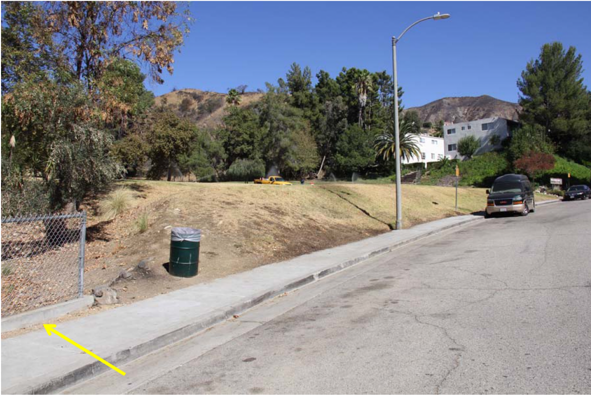
Site 1: Looking northeast across Cabrini Drive West towards Villa Cabrini Park. The yellow arrow points out a culvert inlet structure, which collects and directs runoff away from the park.
