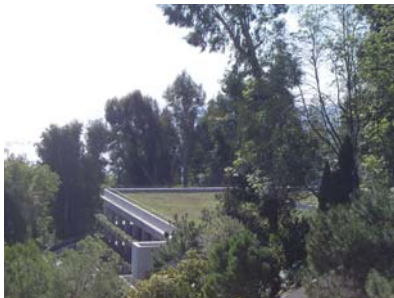
Green roof of a parking structure
