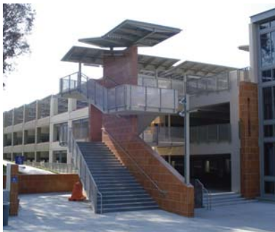
Solar panels on top of parking structure
