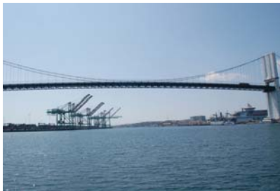
Vincent Thomas Bridge
