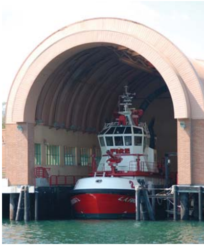
Los Angeles Fire Boat at Port of Los Angeles
