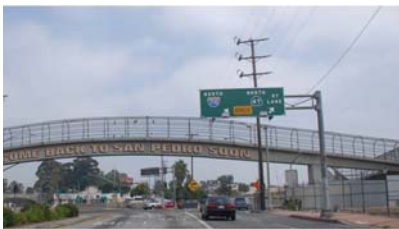
Gaffey Street Pedestrian Bridge
