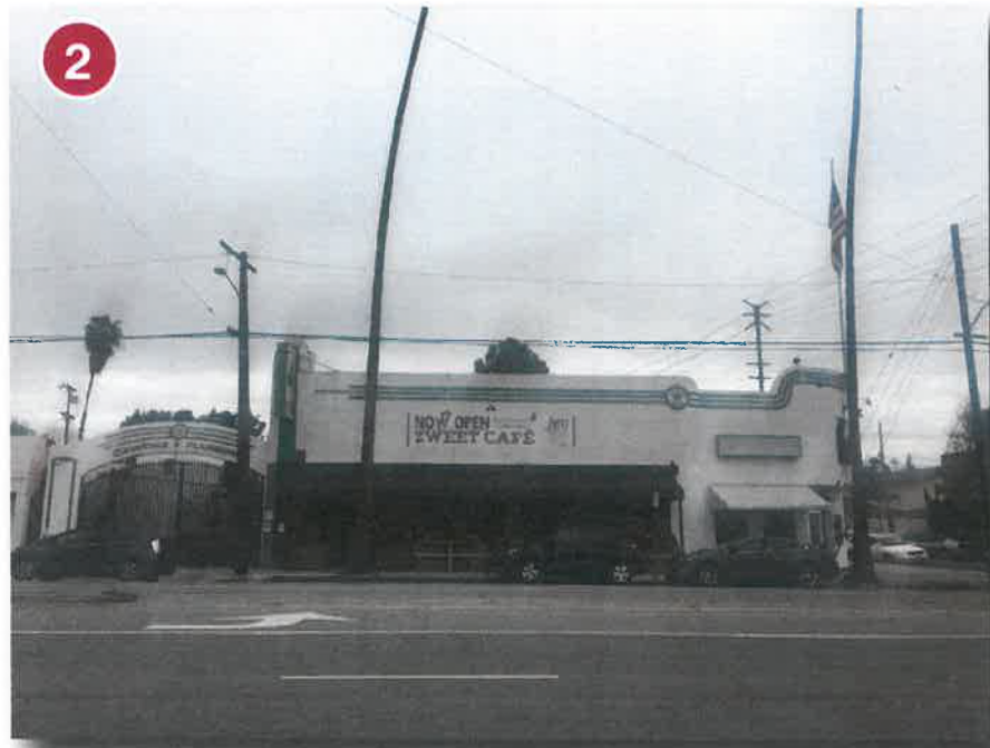
Eagle Rock Blvd, across street facing subject site. Direction: East
