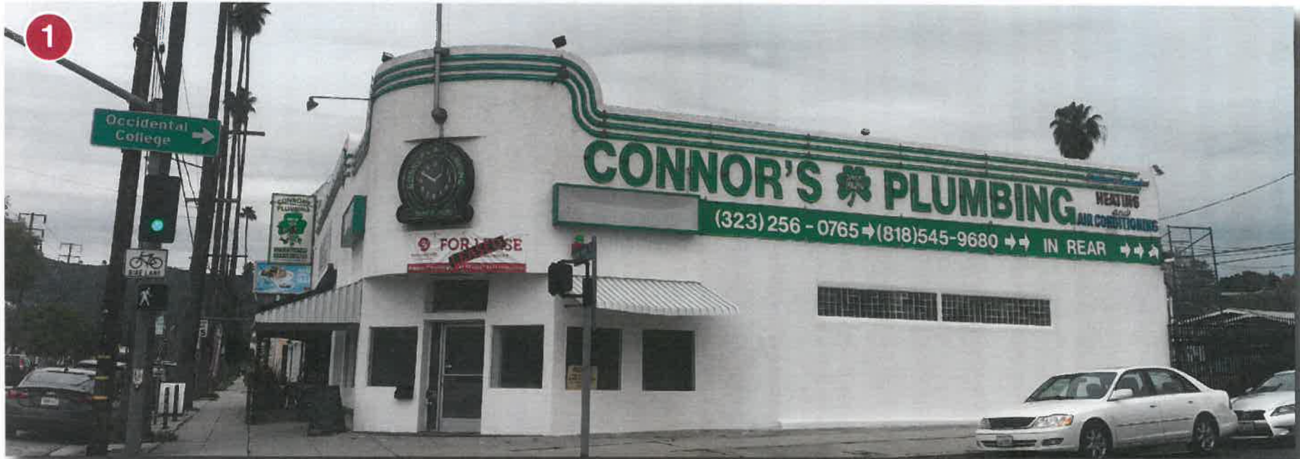
Eagle Rock Blvd & Westdale Ave, across street facing subject site. Direction: Northeast
