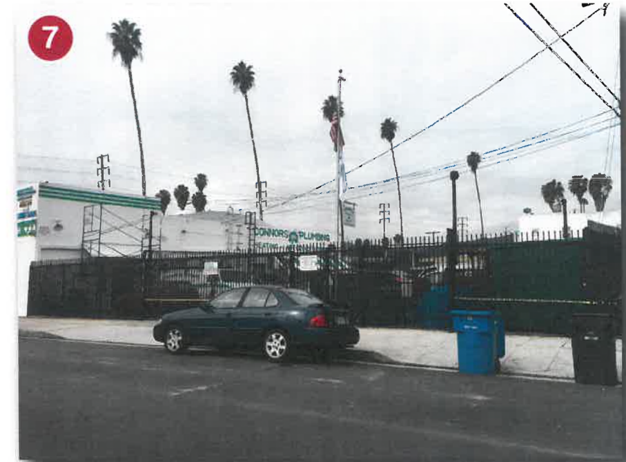
Westdale Ave, across street facing subject site. Direction: Northwest
