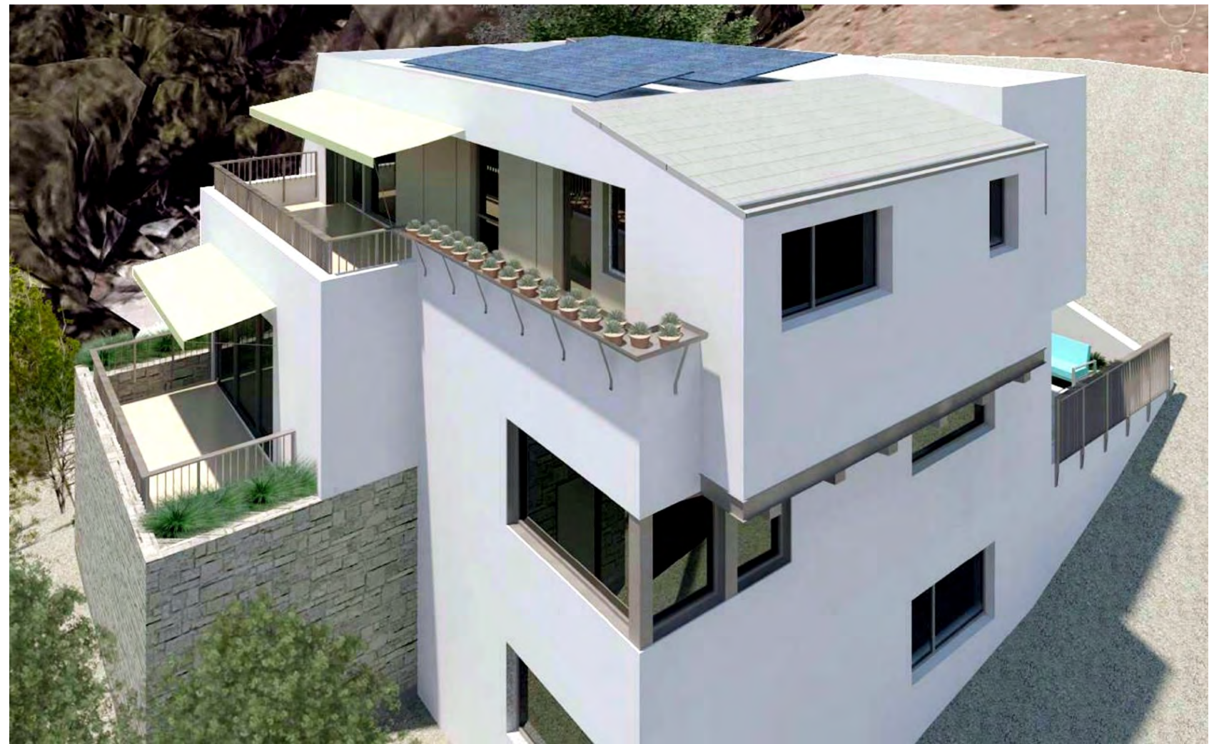
Back Elevation Aerial
