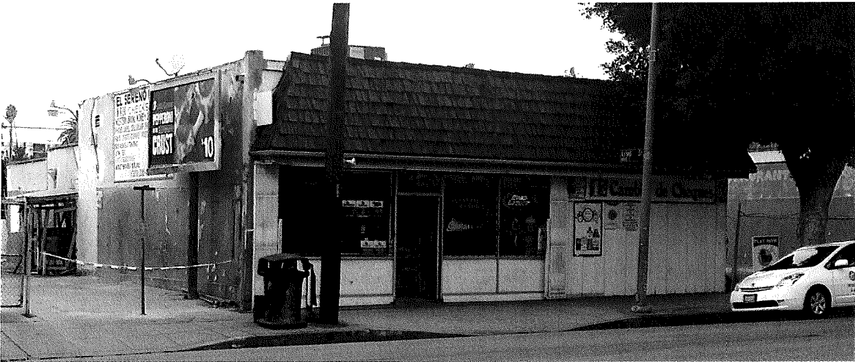
Liquor store east façade
