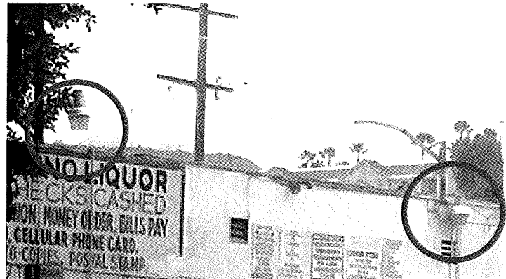
Exterior lighting at parking lot – north wall
