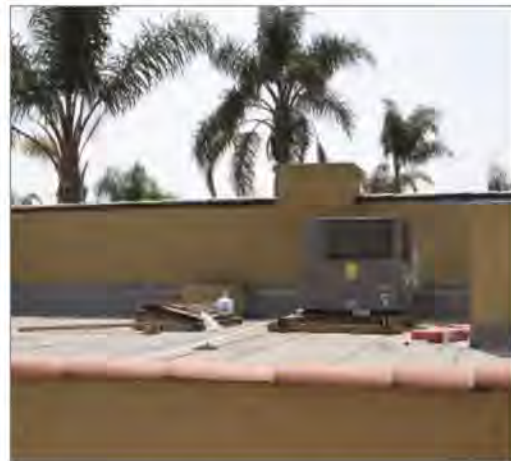
Rooftop mechanical equipment should be placed behind a parapet to screen it from public view.
