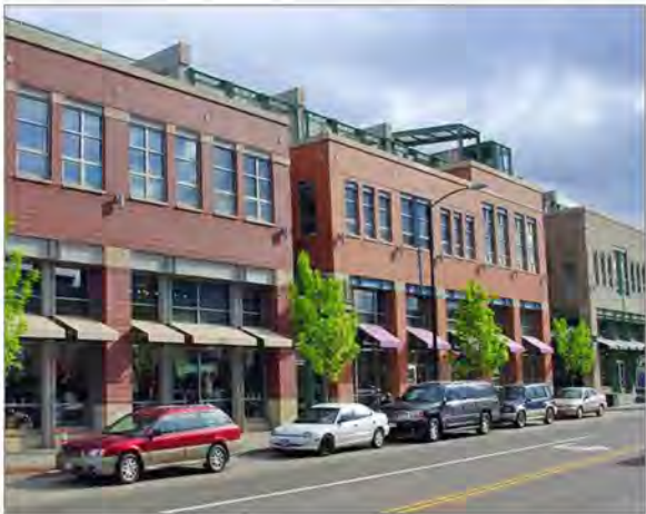
A parking structure "wrapped" by commercial and residential space conceals the parking and allows for windows and Active Floor Area to face the street.
