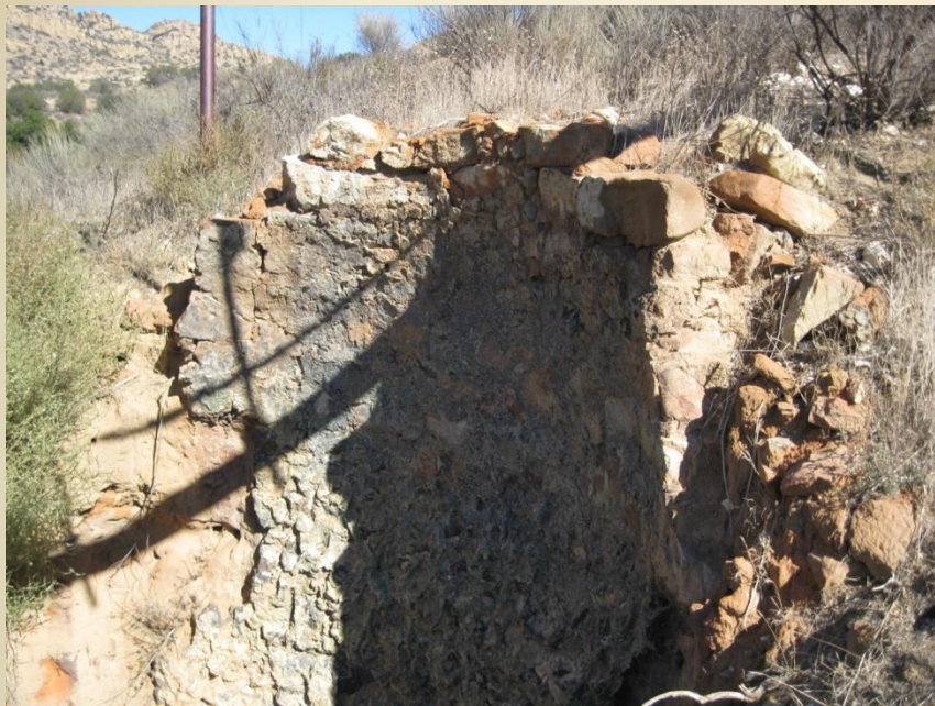
Chatsworth Reservoir limekiln (La Calera) View of back wall, which is all that remains. This kiln is built with hand-hewn sandstone blocks and is over four feet thick; it is at least 18 feet deep
