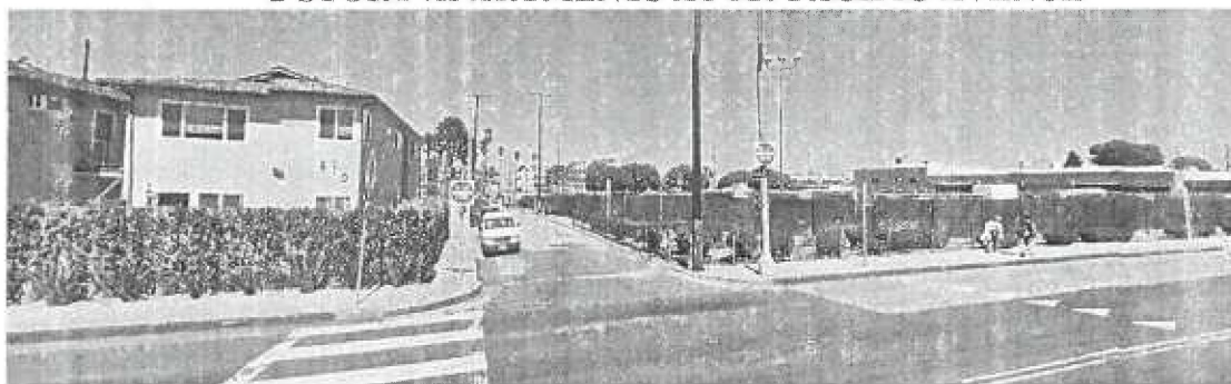
Figure B: 2-STORY APARTMENTS AT 510 PACIFIC AVENUE
