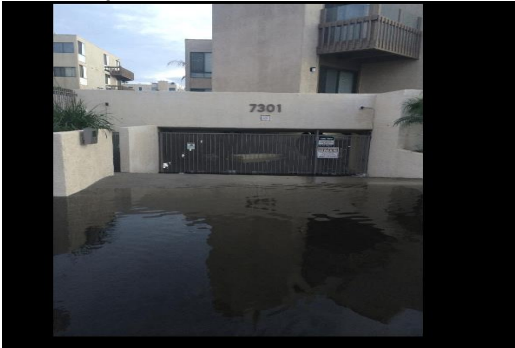
2015 Flood—Mattress floating in City Approved Half Story Underground Garage
