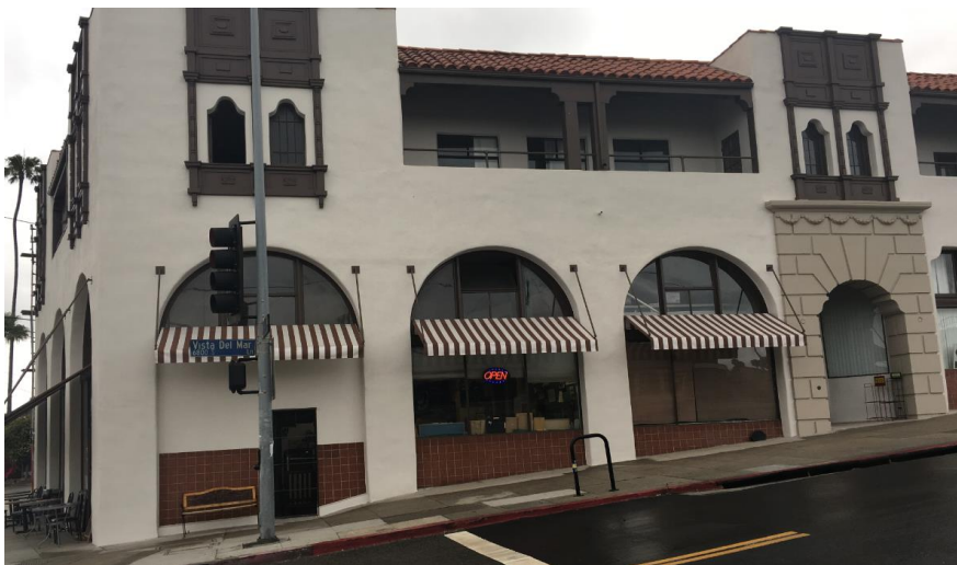
200 Culver Boulevard- applicant's historic building and Tanner's Coffee Shop
