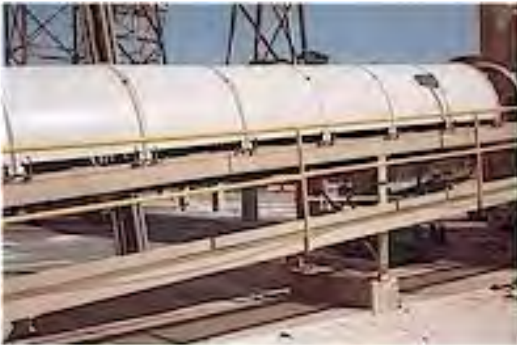
covered conveyor system
