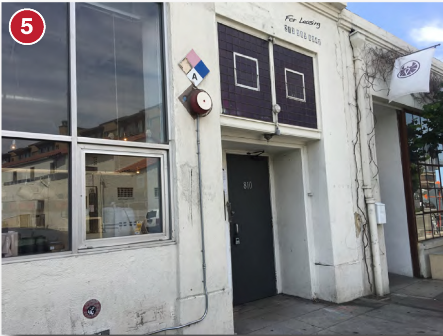
5 E 3rd St, on sidewalk facing subject site. Direction: South
