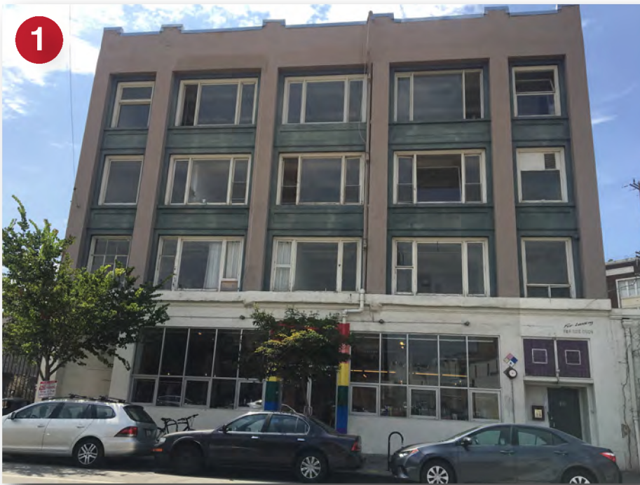
E 3rd St , across street facing subject site. Direction: Southeast
