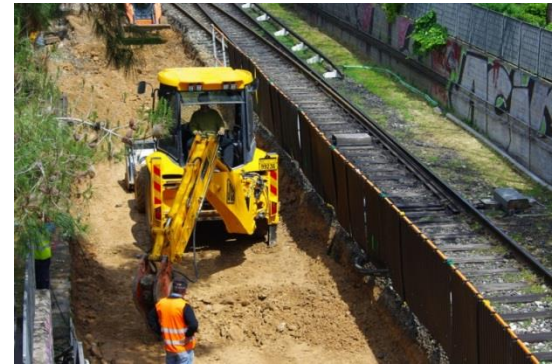
A construction barrier is built at the edge of the site to protect tracks from adjacent work.
