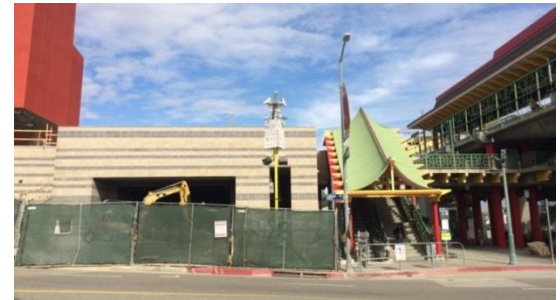
Sidewalk access is blocked for construction project, forcing pedestrians into street or to use less direct paths to the Metro facility.
