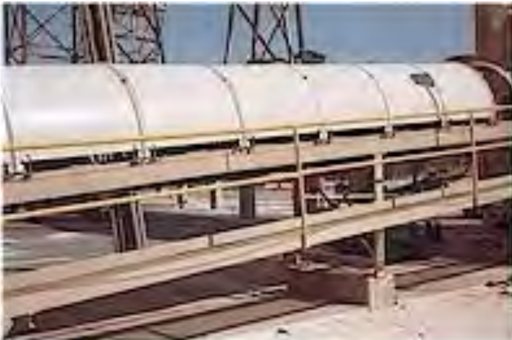
covered conveyor system
