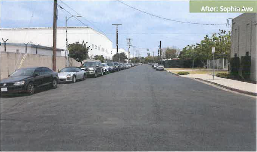
Figure 3 Before and After photos of Sophia Avenue in Council District 12
