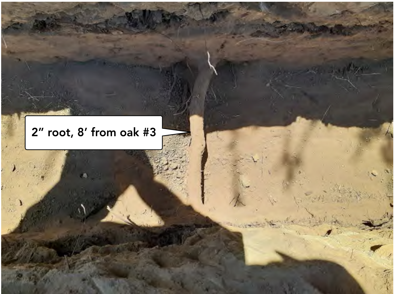
PHOTO 4 - This root is isolated and no more than 2 inches in diameter. Per industry standard, oak tree #3 can be retained if this root is cut at this distance from the trunk, because it is the only root 2 inches or greater in this area. This will allow for the proposed construction to occur while retaining tree #3.
