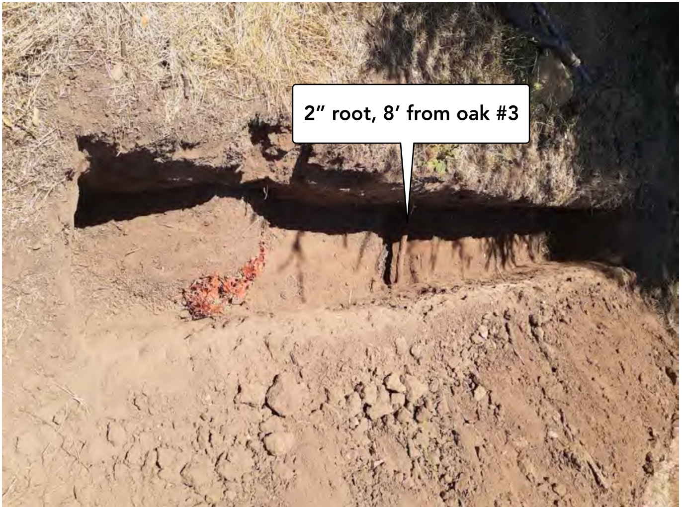
PHOTO 3 - Shows that only one relatively prominent root and very few roots in general were discovered 8 feet away from the trunk of oak tree #3 in this trench. This tree will be minimally impacted by the proposed construction in this area and will be retained.
