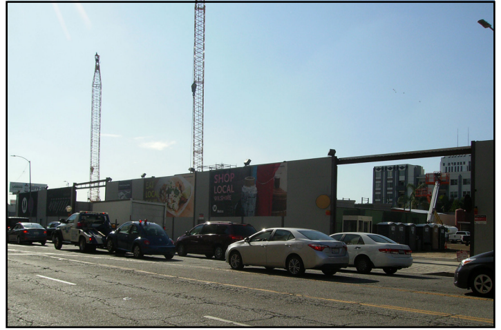
View 7: From the east side of La Brea Avenue, looking southwest at the construction of a Metro Purple Line station.
