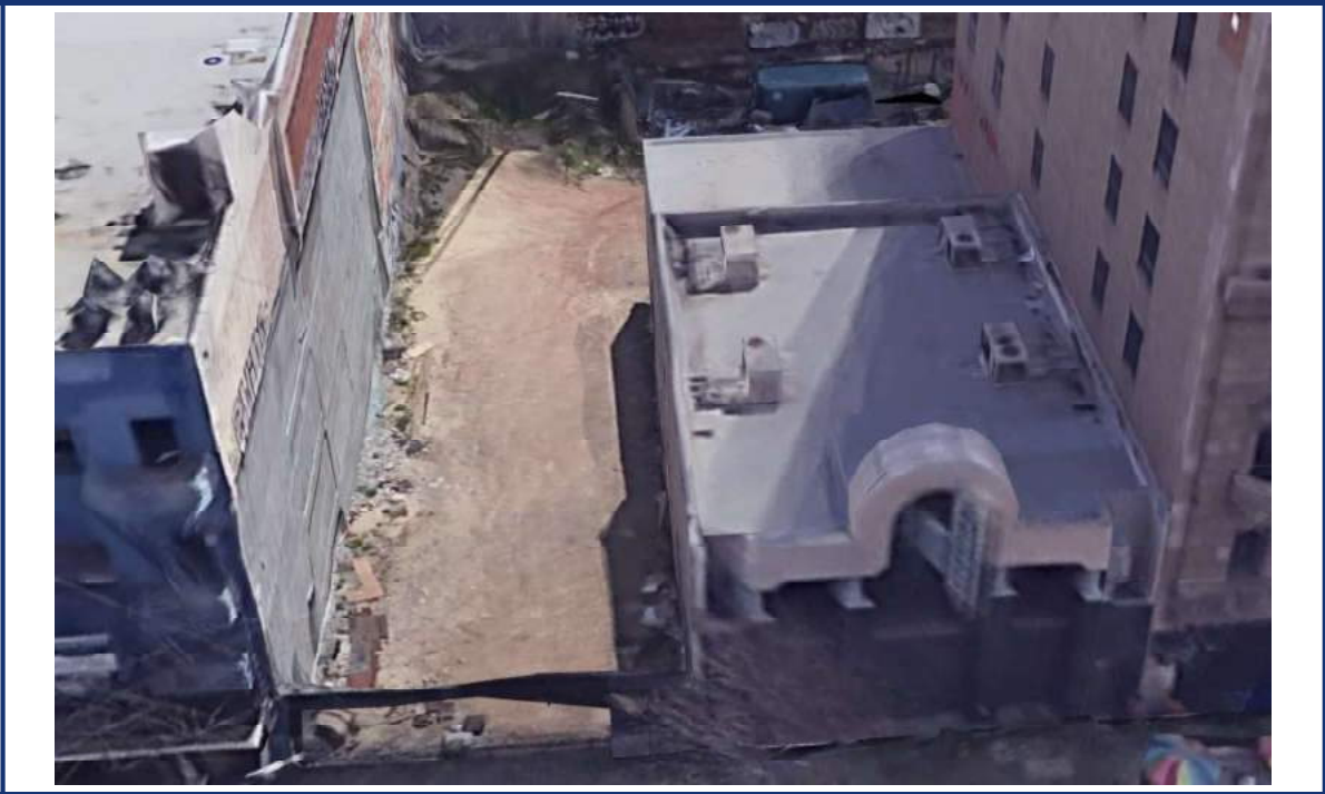
Interior of the site from Hill Street – Google Earth
