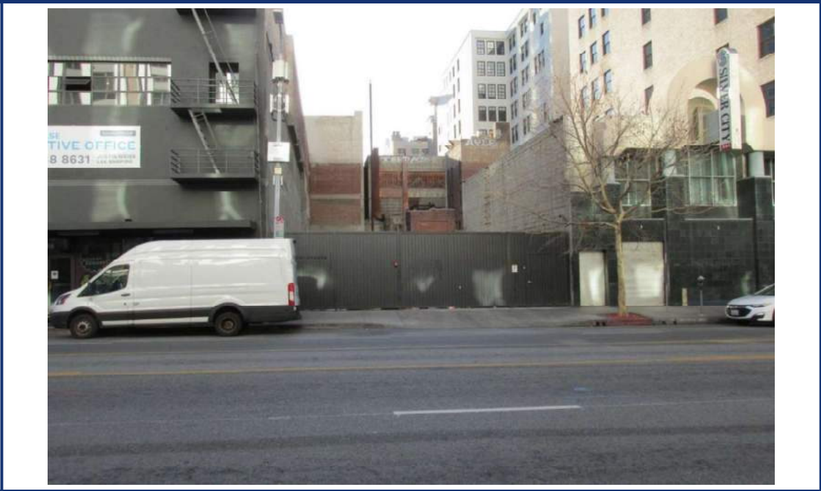
View of the subject from Hill Street – February 3, 2020
