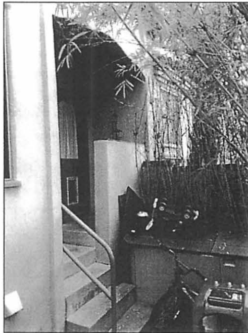
Figure 11. Detail of service entrance on east façade, view north (SWCA, 2019).
