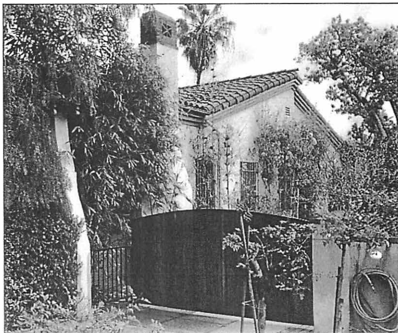
Figure 7. West façade, view southeast (SWCA, 2019).
