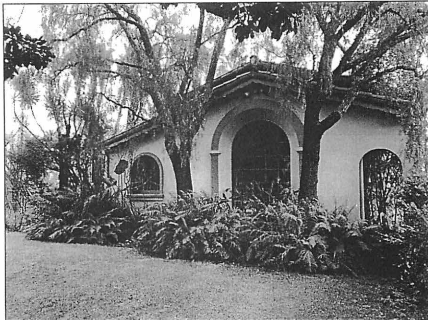
Figure 6. Detail of right side of primary (north) façade, view south (SWCA, 2019).
