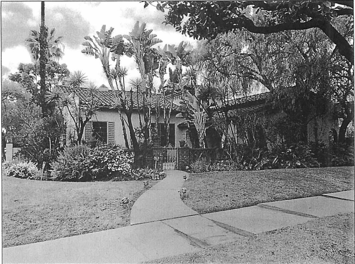
Figure 3. Overview of primary (north) façade of 6500 Olympic Place, view south (SWCA, 2019).
