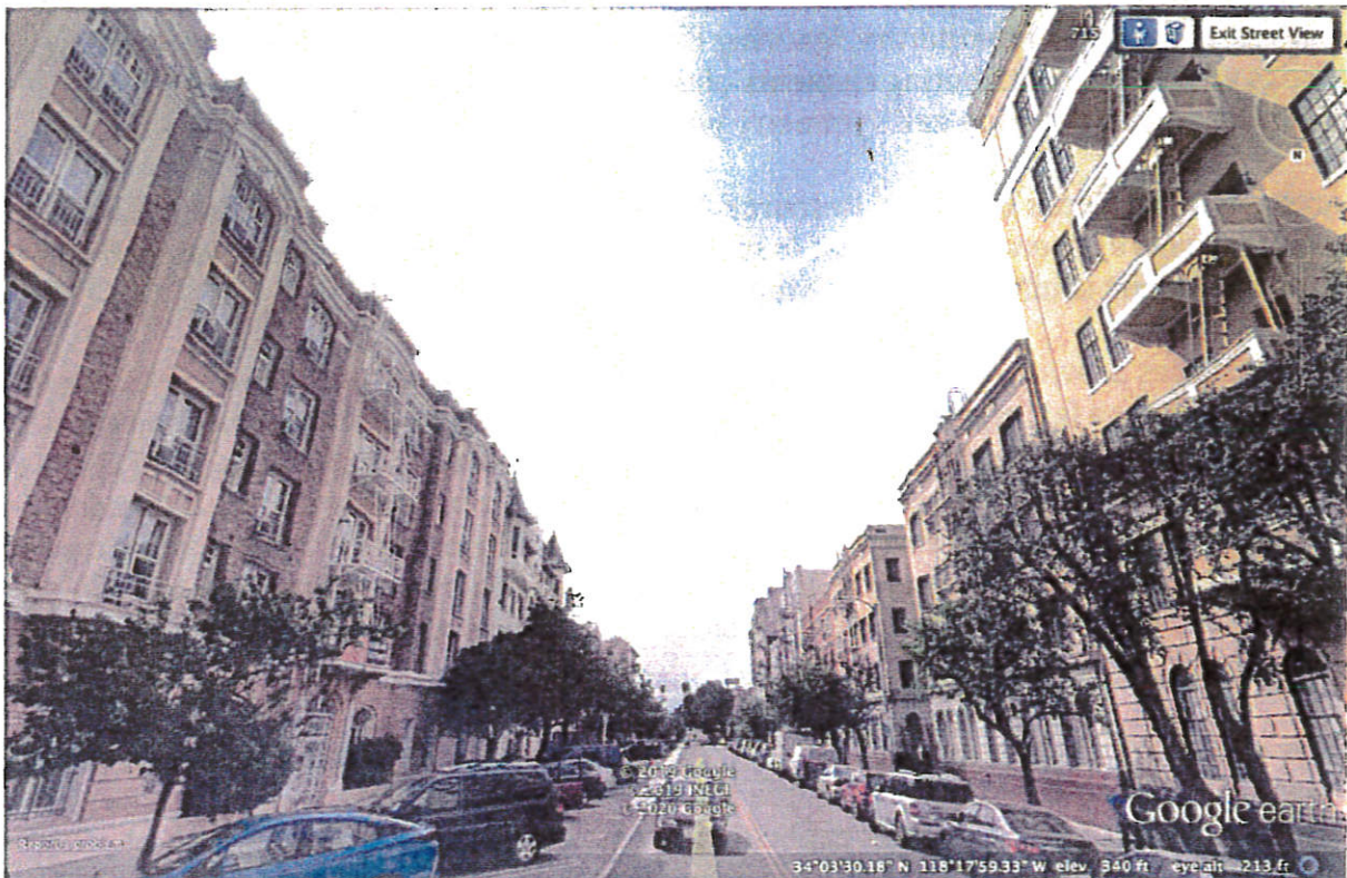
Photo of Project block, showing uniformity of architecture of the District.
