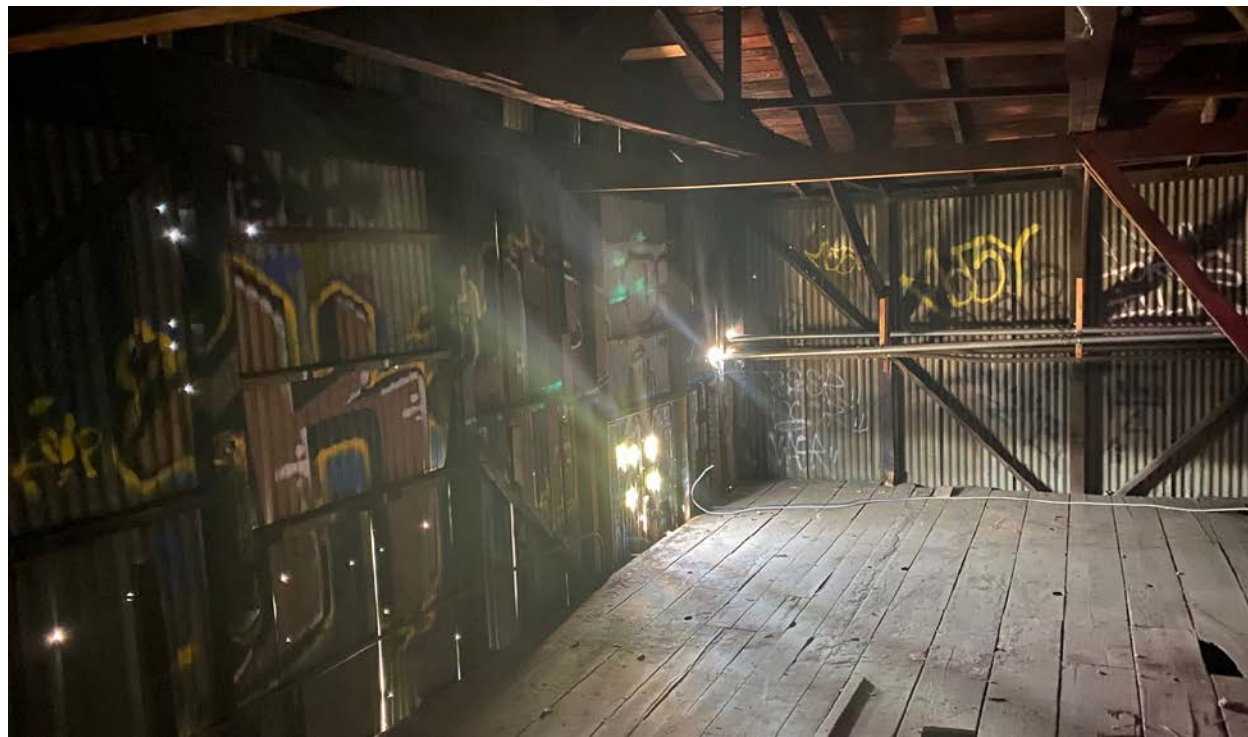
Photograph 7: View of enclosed area subject to habitat assessment and focused surveys for roosting bats.
