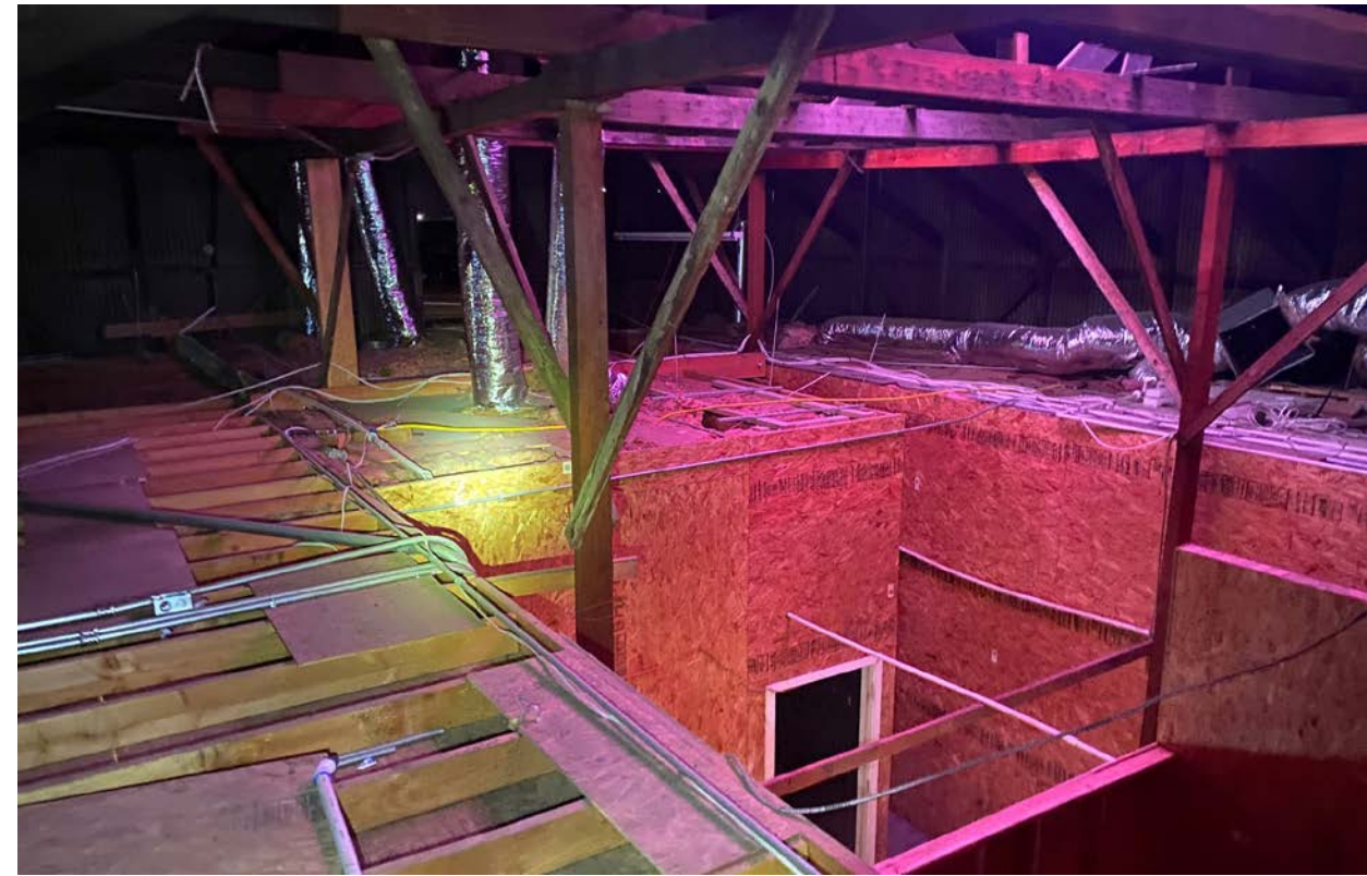
Photograph 6: View of attic area in second building subject to habitat assessment and focused surveys for roosting bats. .
