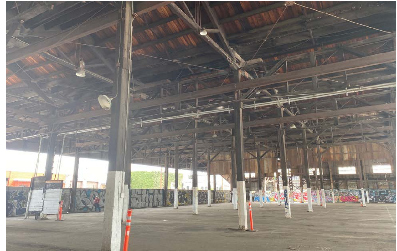
Photograph 2: View of ceiling with support columns, ceiling joists, braces and other surfaces examined for bat roosts.
