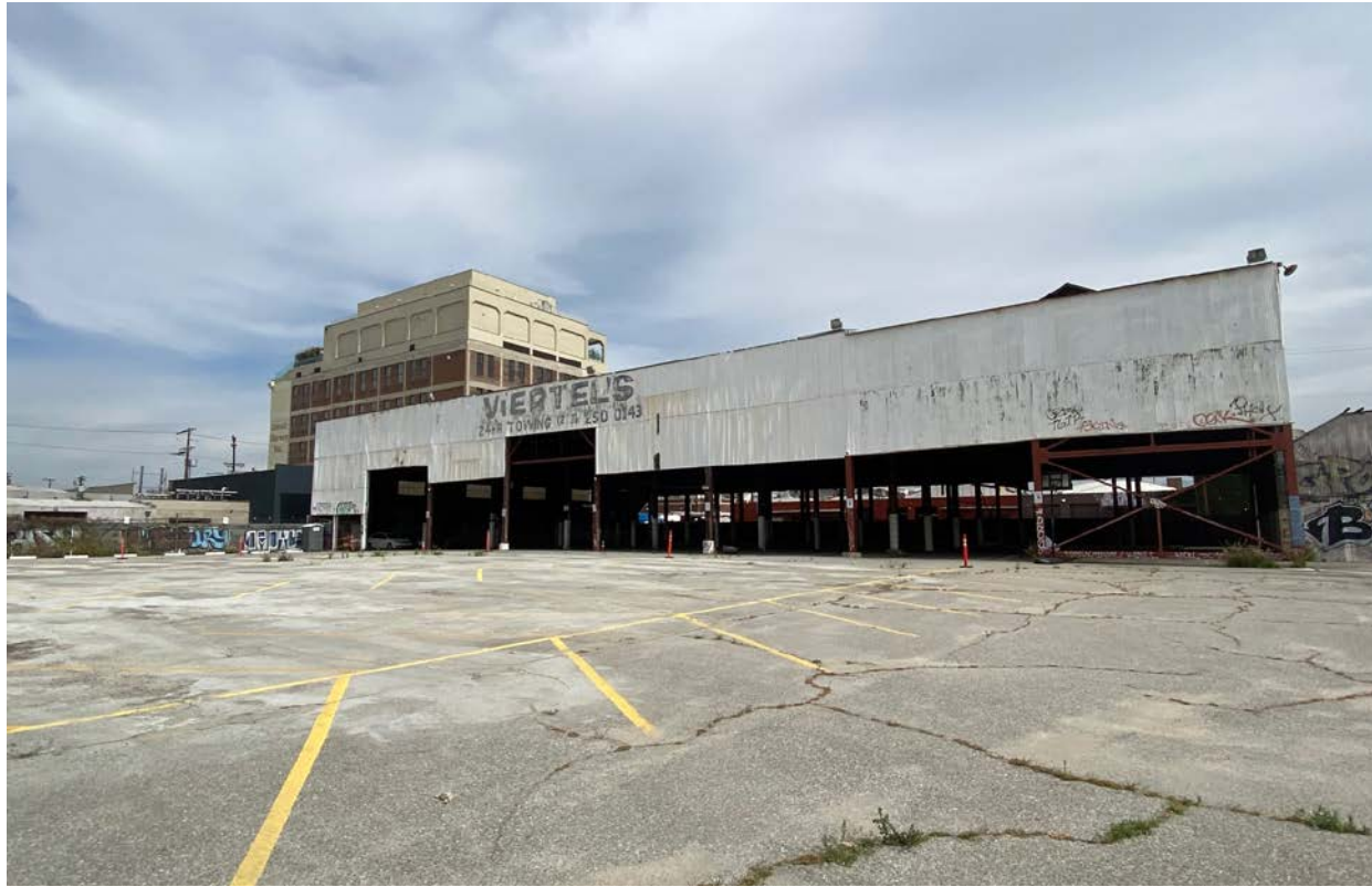
Photograph 1: View of Building subject to habitat assessment and focused surveys for roosting bats.
