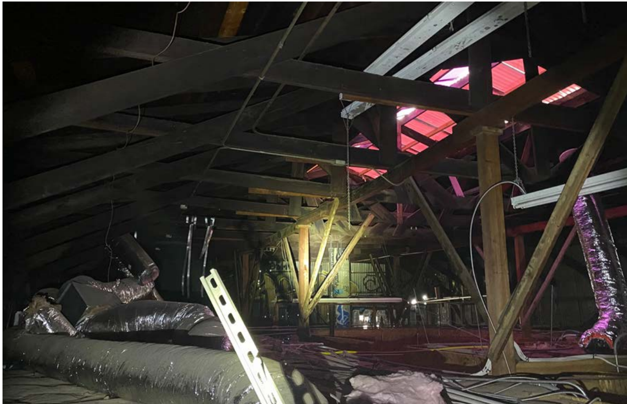
Photograph 5: View of attic area subject to habitat assessment and focused surveys for roosting bats.
