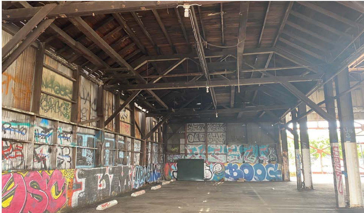
Photograph 3: View of ceiling with support columns, ceiling joists, braces and other surfaces examined for bat roosts.
