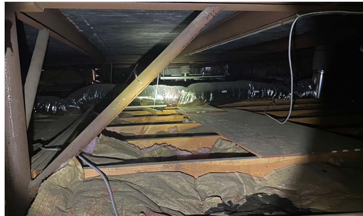
Photograph 8: View of attic area subject to habitat assessment and focused surveys for roosting bats.
