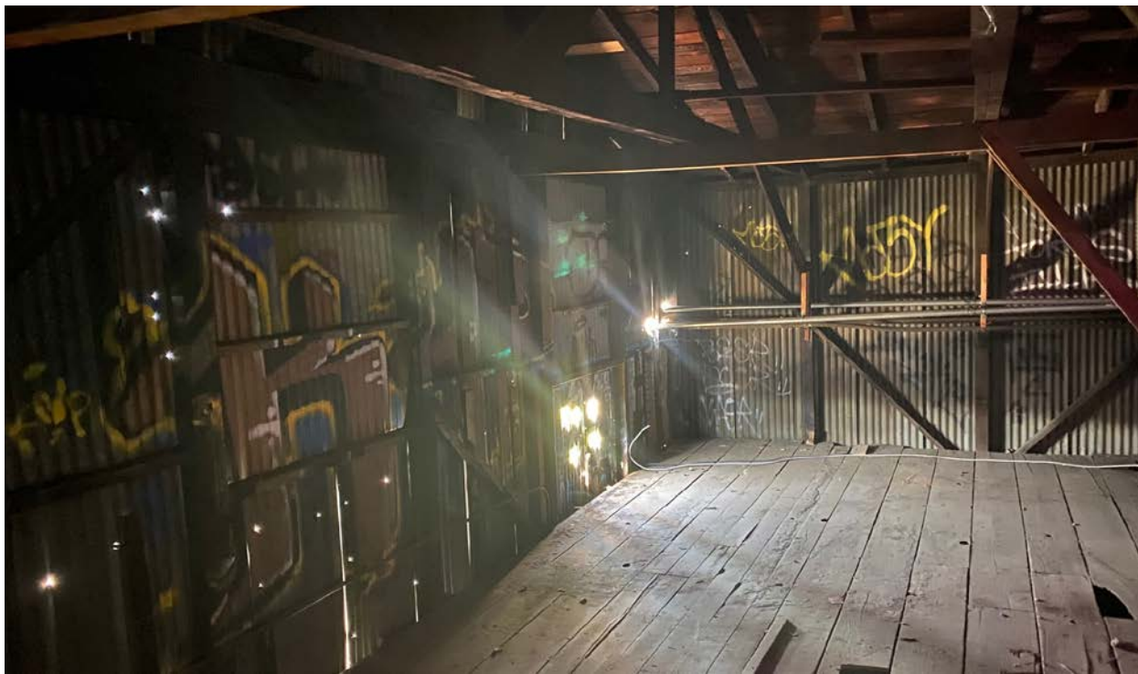
Photograph 7: View of enclosed area subject to habitat assessment and focused surveys for roosting bats.
