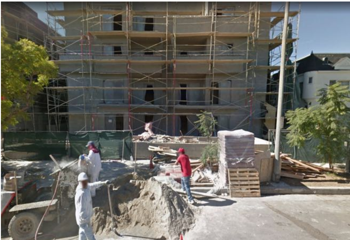
Building "Hayworth Hyde."
