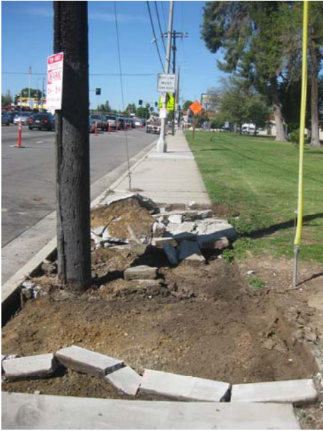
Demolished Sidewalk CD 3 – Reseda Park & Recreational Center
