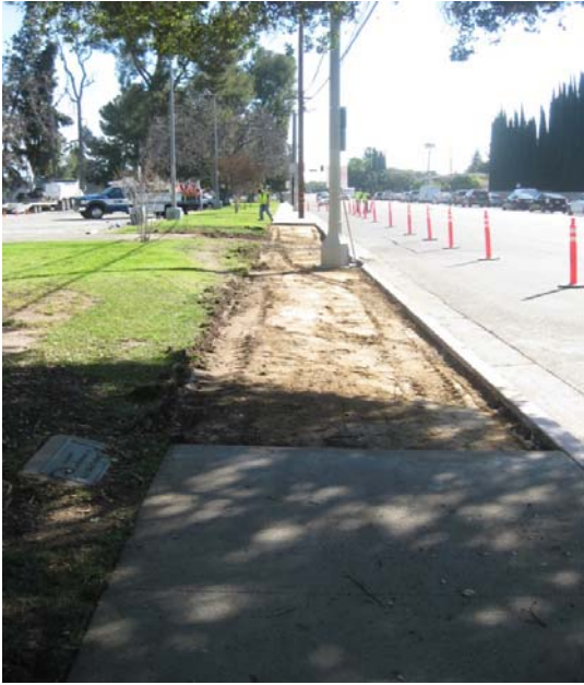
Demolished Sidewalk CD 3 – Reseda Park & Recreational Center
