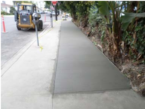
New Sidewalk CD 11 – West LA Municipal Building
