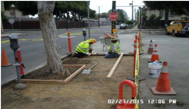
Forming for Concrete Placement CD 11 – West LA Municipal Building
