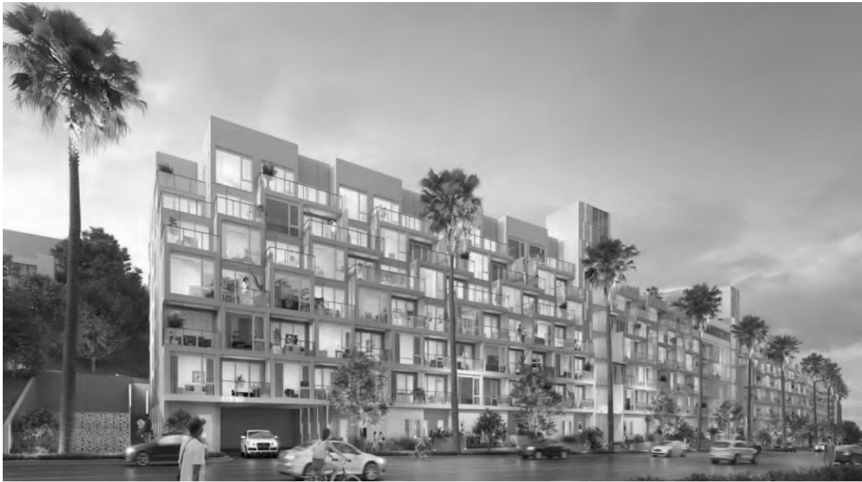
Figure 3. One of the proposed buildings of the project, showing a lengthy barrier to bird flights, and abundant glass and interior lighting, both features of which increase bird-window collision risk. The image is from https://la.urbanize.city/post/mixed-use-project-inches-forward-1185-w-sunset-boulevard-echo-park .
